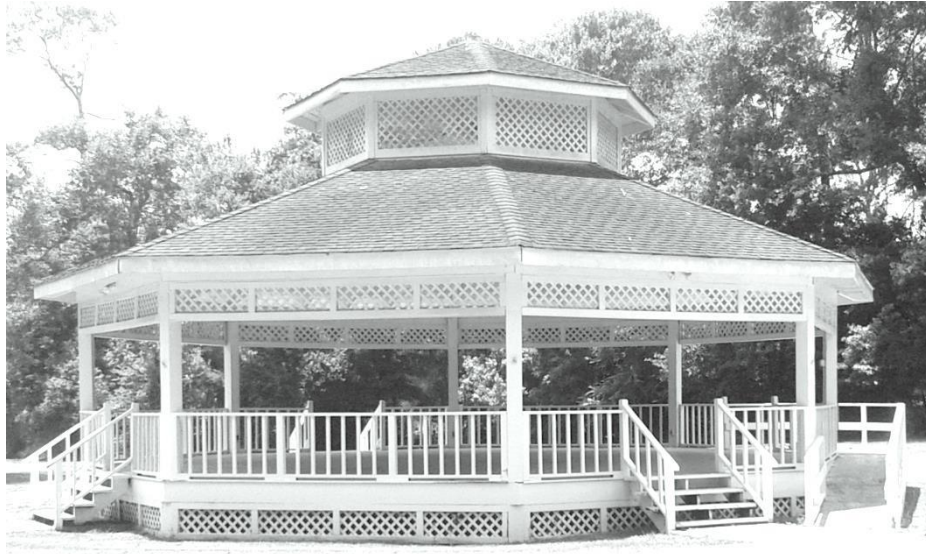
Gazebo (with electricity)
